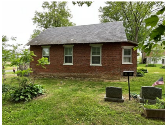
Photo 5. View to east, west (side) elevation.
