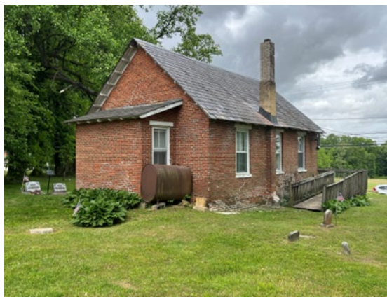
Photo 7. View to northwest.
