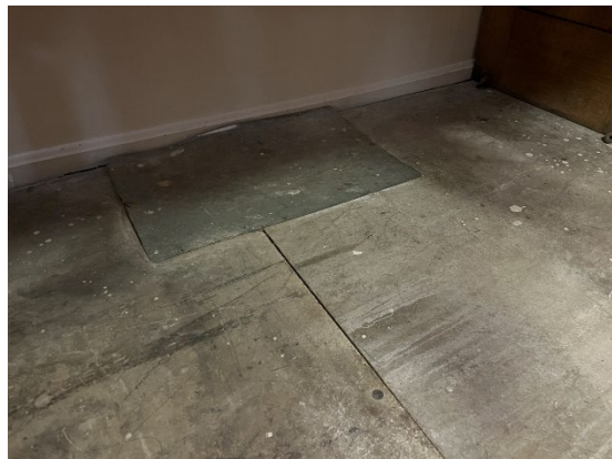
Photo 14. Detail view of floor at northeast corner of Sanctuary.
