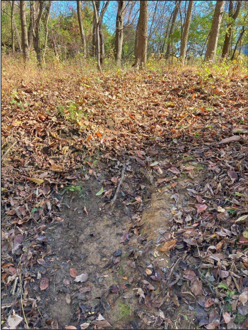
Figure 17. Detail of erosion on cutbank, revealing subsoil
