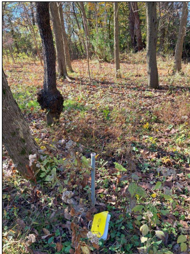
Figure 14. Potential monitoring well encountered within the vicinity of the cemetery, with notebook for scale (View to south).
