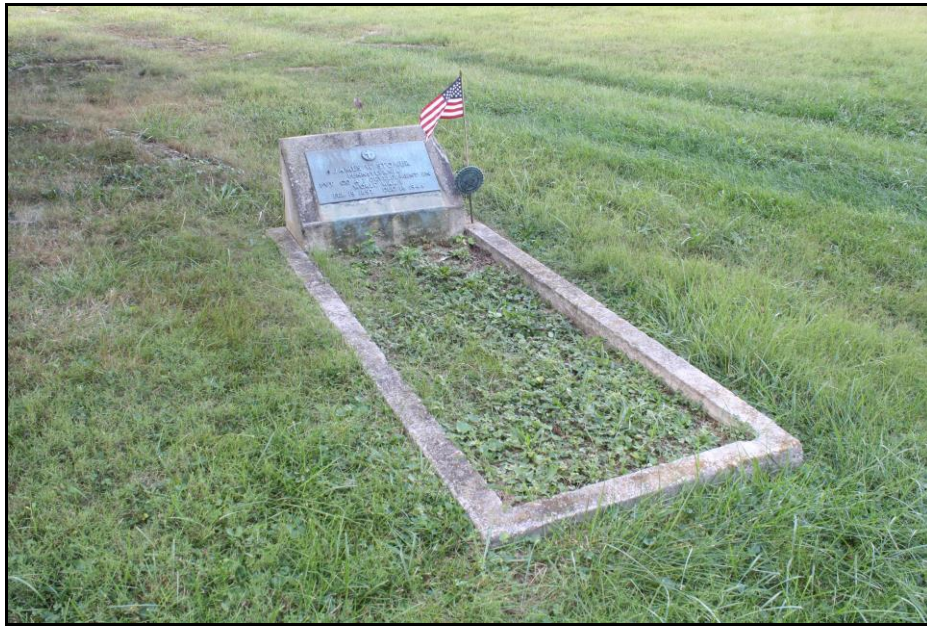
Figure 27: Cast concrete slant-front marker with bronze plaque and cast concrete plot enclosure for James Stoner (d. 1944) who served in World War I; Photo view: South; Photographer: Jason Harpe; Date: September 19, 2023.
