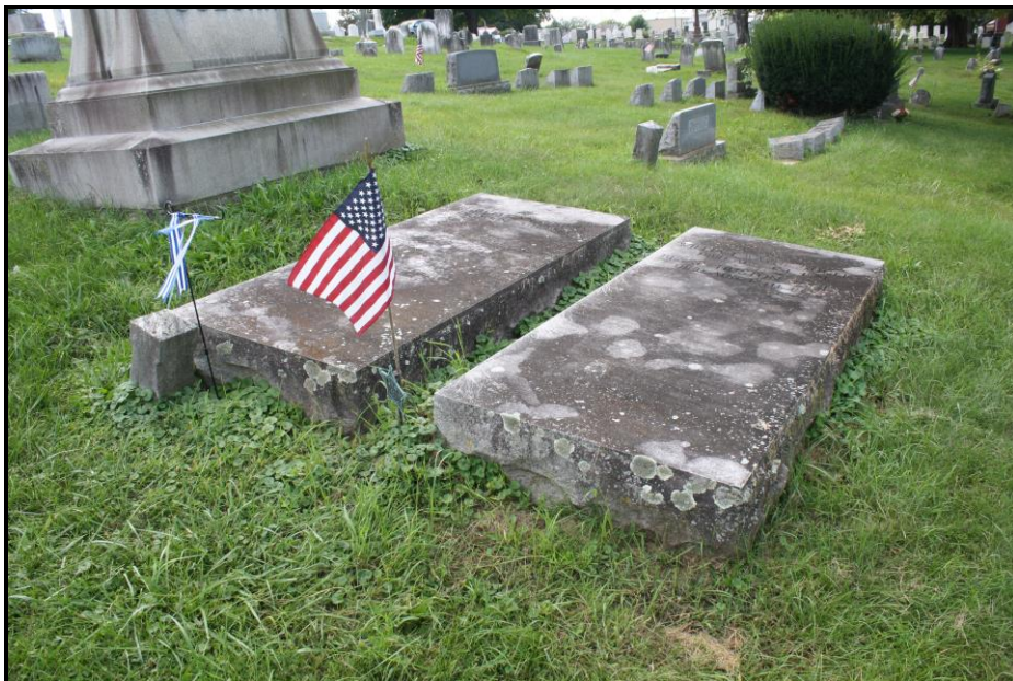
Figure 60: Biofilm and lichens on Rogers family ledger stones; Photo view: West; Photographer: Jason Harpe; Date: September 20, 2023.
