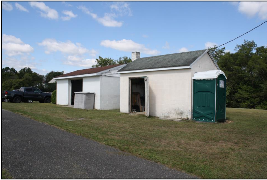
Figure 10: Concrete block storage buildings at Mt. Vernon/Lebanon Cemetery; Photo view: Northwest; Photographer Jason Harpe; Date: September 19, 2023.
