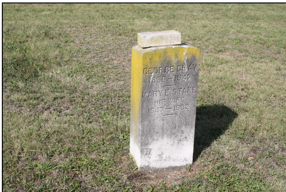
Figure 39: Marble gravemarker for George Cray (1856-1942) and his wife, Mary E. Stake Cray (1847-1932) showing atmospheric staining and biological growth. Photo view: West; Photographer: Jason Harpe; Date: September 19, 2023.
