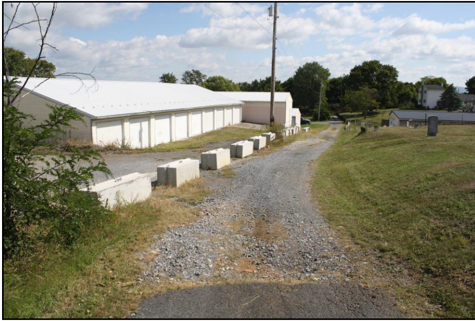
Figure 16: One-lane, paved road that extends from Mt. Vernon/Lebanon Cemetery’s northeast corner to an unnamed road that leads to Lincoln Way Road. Chambersburg Storage Rentals units are visible at this elevation; Photo view: East; Photographer Jason Harpe; Date: September 19, 2023.
