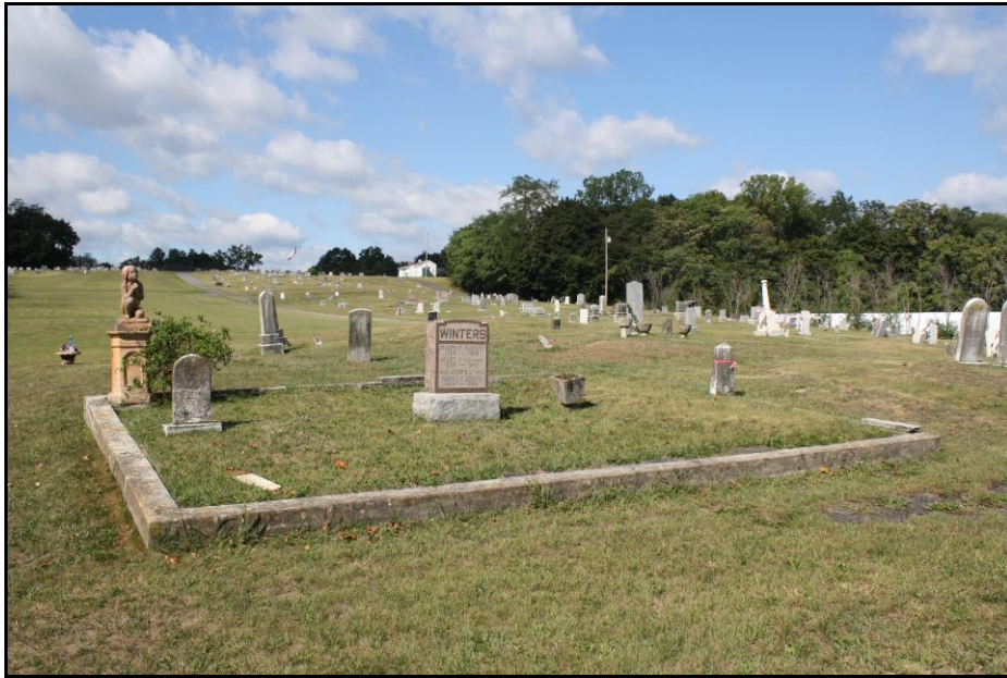
Figure 33: Cast concrete plot enclosure for the Winters family; Photo view: West; Photographer Jason Harpe; Date: September 19, 2023.
