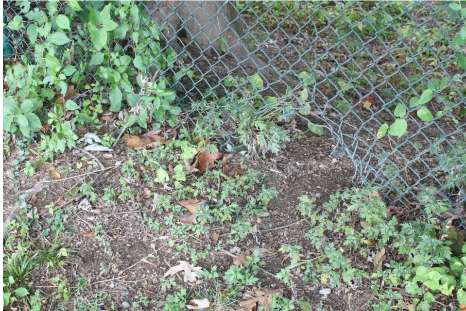
Figure 42: Damage to the chain link fence at Lincoln Cemetery's east elevation; Photo view: East; Photographer: Jason Harpe; Date: September 18, 2023.
