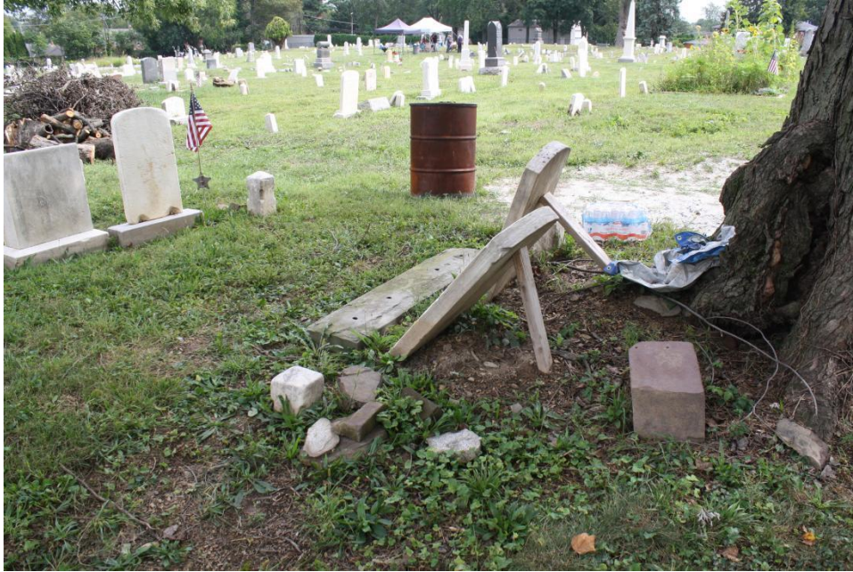
Figure 51: Displaced marble tablets; Photo view: South; Photographer: Jason Harpe; Date: September 18, 2023.
