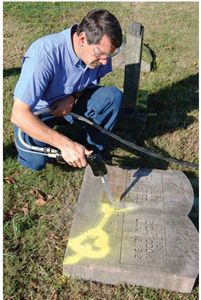
Figure 18. Graffiti is carefully removed using a low-pressure dry-ice misting instrument. Photo: Jason Church.
