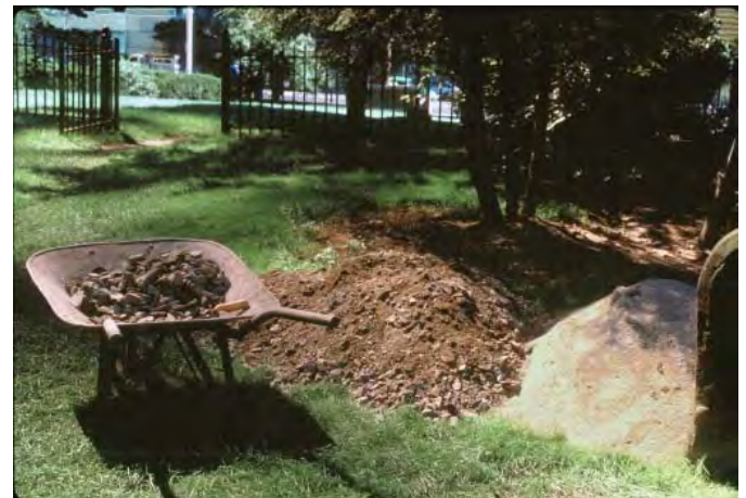
Figure 20b. To facilitate drainage, crushed stone, gravel, and sharp sand line the hole and are hand-tamped around the stone after placement. Photo: Fran Gale.
