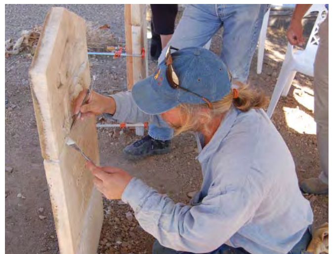
Figure 21. Cracks in a stone marker should be filled to keep water and debris out and prevent the crack from becoming larger. A patching mortar is designed to be used, in this case, with historic marble. Photo: Mary Striegel.
