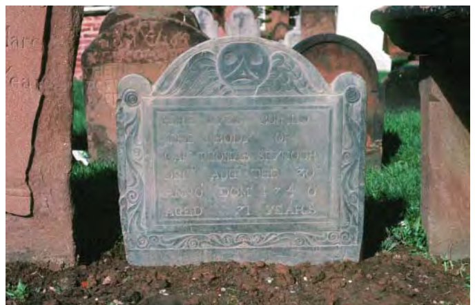
Figure 20c. The reset ground-supported grave marker should be level and plumb. Photo: Fran Gale.
