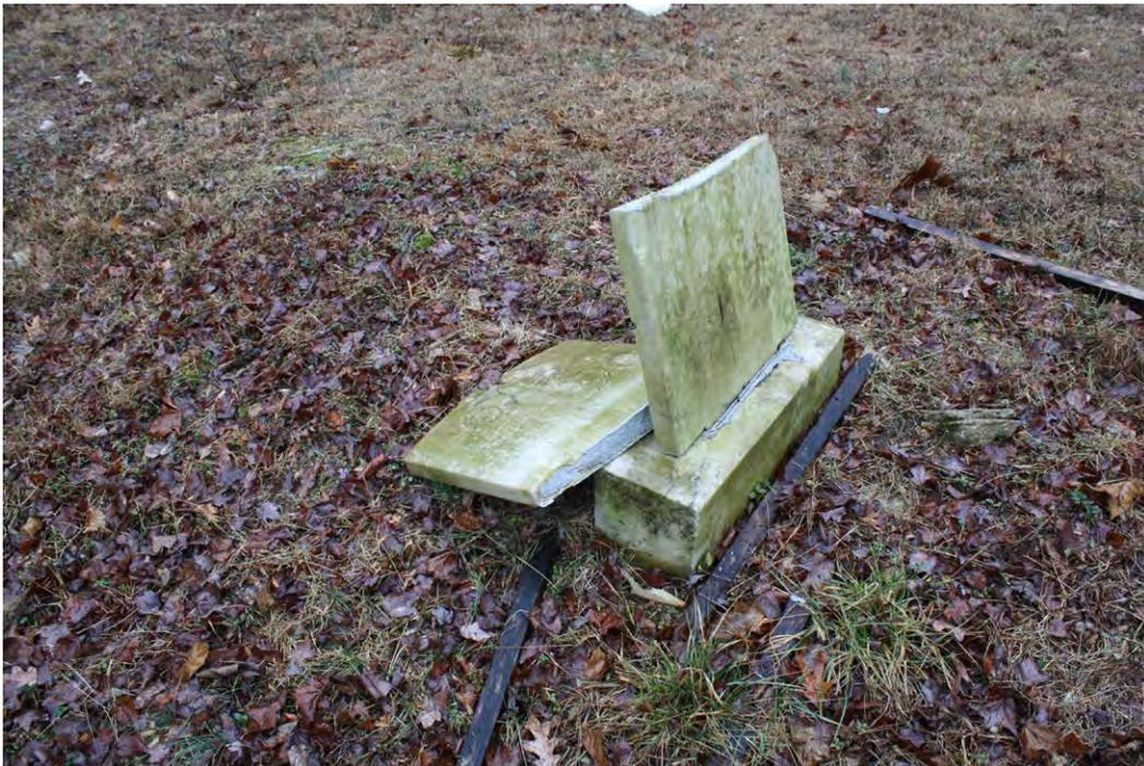
Figure 3.8: Damaged marble tab-in-socket with previous inappropriate repairs
