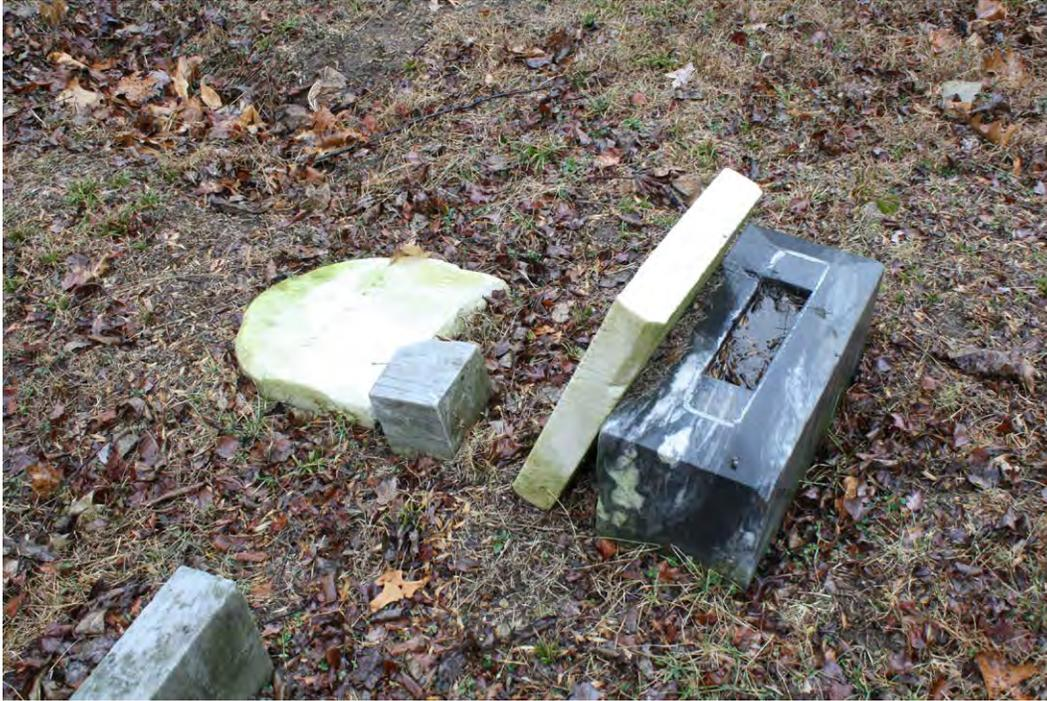
Figure 3.7: Damaged marble tablet with a granite base at the Lindley Hill Cemetery.
