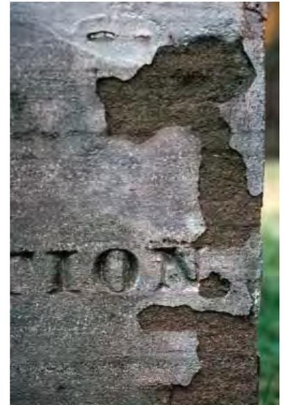
Figure 14. High-pressure water washing can damage grave markers. The photograph shows "wand marks" on the headstones produced by inappropriate pressure washing. Photo: Jason Church.
