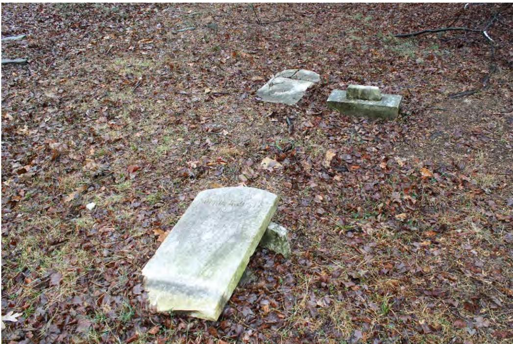
Figure 3.6: Damaged marble ground-supported tablet and tab-in-socket gravemarkers
