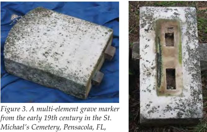
Figure 3. A multi-element grave marker from the early 19th century in the St. Michael’s Cemetery, Pensacola, FL, consists of a vertical element with tabs (left image) into a slotted base (right image). Photo: Fran Gale.
