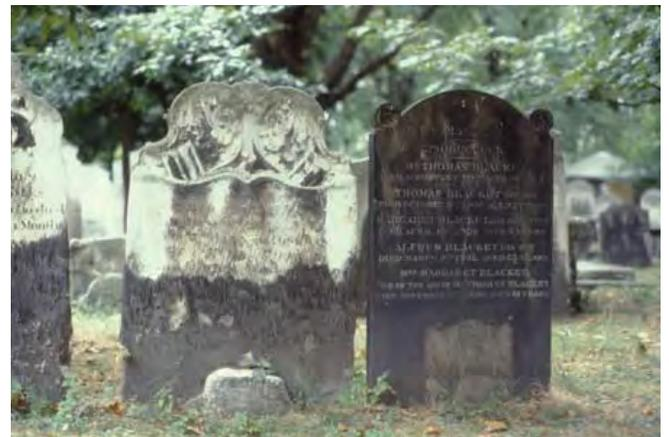
Figure 9. The limestone and sandstone grave markers in this historic cemetery have different weathering processes. On the left, the limestone shows surface loss in areas exposed to rainwater and gypsum crust formation below. The sandstone marker on the right displays uniform soiling, but surface hardening may be occurring. Photo: Fran Gale.
