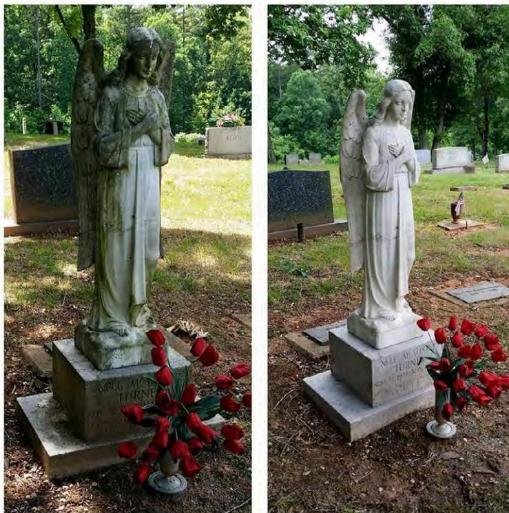
Figure 4.15: Before-and-after photographs of a marble angel in Lincolnton, North Carolina, after being cleaned with D/2 Biological Solution.
