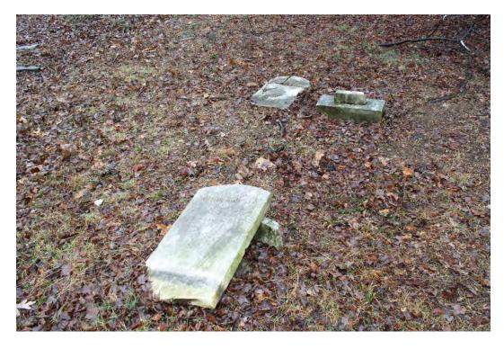
Figure 3.6: Damaged marble ground-supported tablet and tab-in-socket gravemarkers at the Lindley Hill Cemetery.
