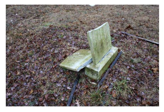
Figure 3.8: Damaged marble tab-in-socket with previous inappropriate repairs at the Lindley Hill Cemetery.
