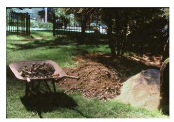
Figure 20b. To facilitate drainage, crushed stone, gravel, and sharp sand line the hole and are hand-tamped around the stone after placement. Photo: Fran Gale.
