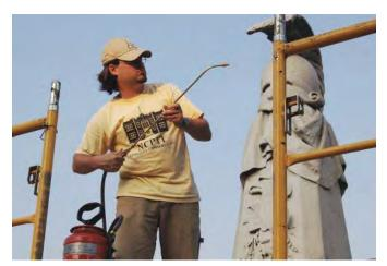
Figure 24. A severely deteriorating monument or grave marker can be treated with a stone consolidant. The treatment is usually applied using a spray system. The consolidant soaks into the stone and replaces mineral binders that hold the stone together. On-site and laboratory testing and evaluation are performed prior to using this non-reversible type of treatment. Photo: Lucas Flickinger.
