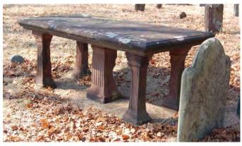
Figure 4. This sandstone table tomb, located in Cedar Grove Cemetery, New London, CT, is an engineered grave marker structure consisting of a horizontal stone tablet supported by four vertical table "legs" with and a central column, Photo: Jason Church.
