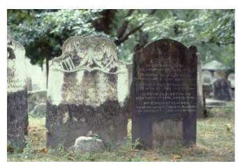
Figure 9. The limestone and sandstone grave markers in this historic cemetery have different weathering processes. On the left, the limestone shows surface loss in areas exposed to rainwater and gypsum crust formation below. The sandstone marker on the right displays uniform soiling, but surface hardening may be occurring. Photo: Fran Gale.
